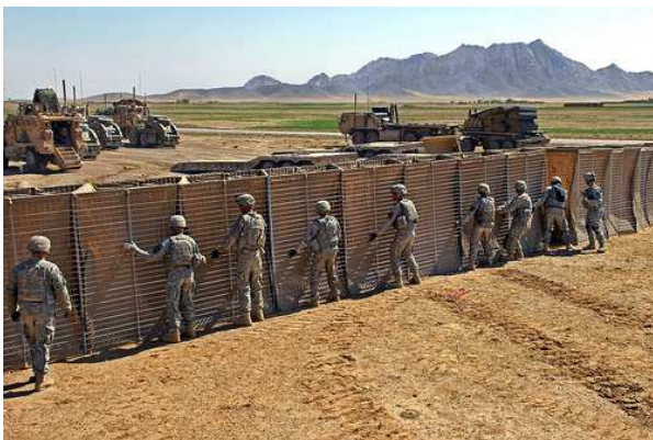
Checkpoint construction in Robat, Afghanistan, March 2010 – photo credit: US Army/flickr
